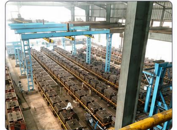
Automatic Sand Plant 30 MT/HR Sand Handling System
