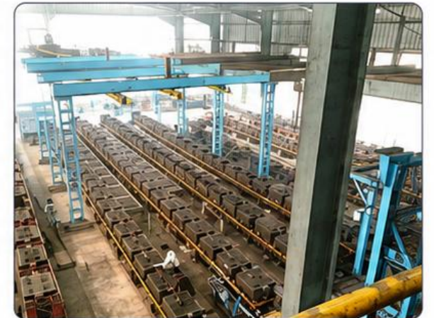
Automatic Sand Plant 30 MT/HR Sand Handling System
